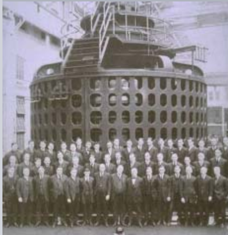
Huge waterwheel generators destined for Niagara Falls and other hydro generating stations were manufactured in the building where gas turbines are assembled today.
